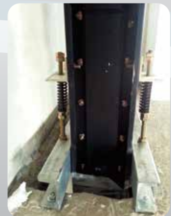
Vertical Spring Hanger (side view)
