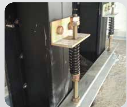
Vertical Spring Hanger (front view)
